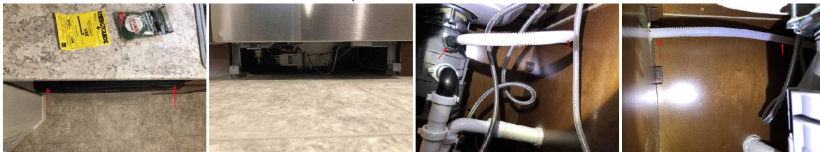
Method 2-High drain loop with waste tee or disposer
